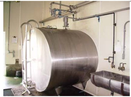
The bulk tank goes through the wall. It is made of stainless steel and is kept spotless inside and out!
